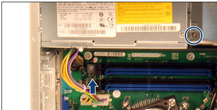
Figure 25: Disconnecting power cable
