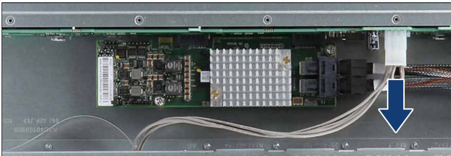
Figure 65: Disconnecting power cable from the HDD backplane
