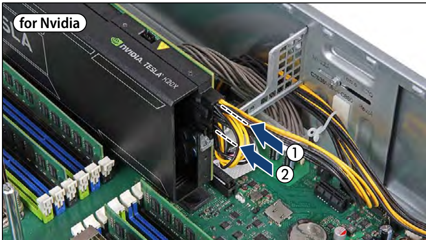
Figure 294: Cabling the primary GPGPU card (Nvidia)
