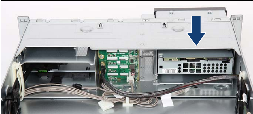
Figure 320: Installing LTO drive
