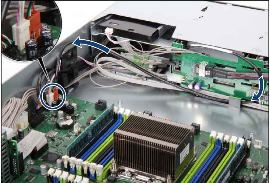
Figure 196: Installing the tape/RDX drive
