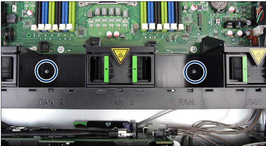
Figure 71: Installing the fan box
